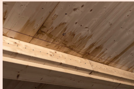
Building damage through wetness
