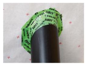
Image shows Rissan sealing the internal membrane (Majpell or Majrex) to the penetration.
