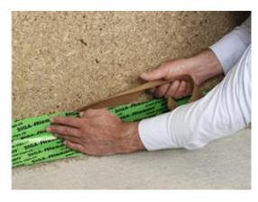
Rissan 100 or 150 mm wide, combined with the primer SIGA Dockskin is the perfect solution for permanently airtight bonding of wall elements to floor and ceiling on the inside.
