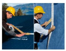
Wigluv is Europe's leading external façade sealing tape and the optimum solution for permanently windtight sealing of breathable membranes and facade membranes, for overlaps, penetrations and bonding the membrane to the concrete slab edge on the outside.
