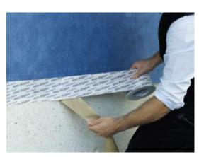
The image shows 150 sealing the membrane Majvest to the slab edge.
