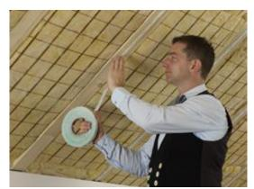
Image showing the quick installation of vapour control layers without the need for mechanical fastening such as a stapler.
