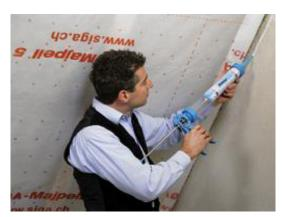
Image shows Primur being laid via cartridge carrier to hard substrate for airtight bonding of Majpell membrane.
