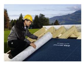
Majcoat is Europe's leading external weatherproof roof and wall membrane. The driving rain-proof and diffusion-open breathable membrane Majcoat is specified for creating a permanently windtight building envelope.
